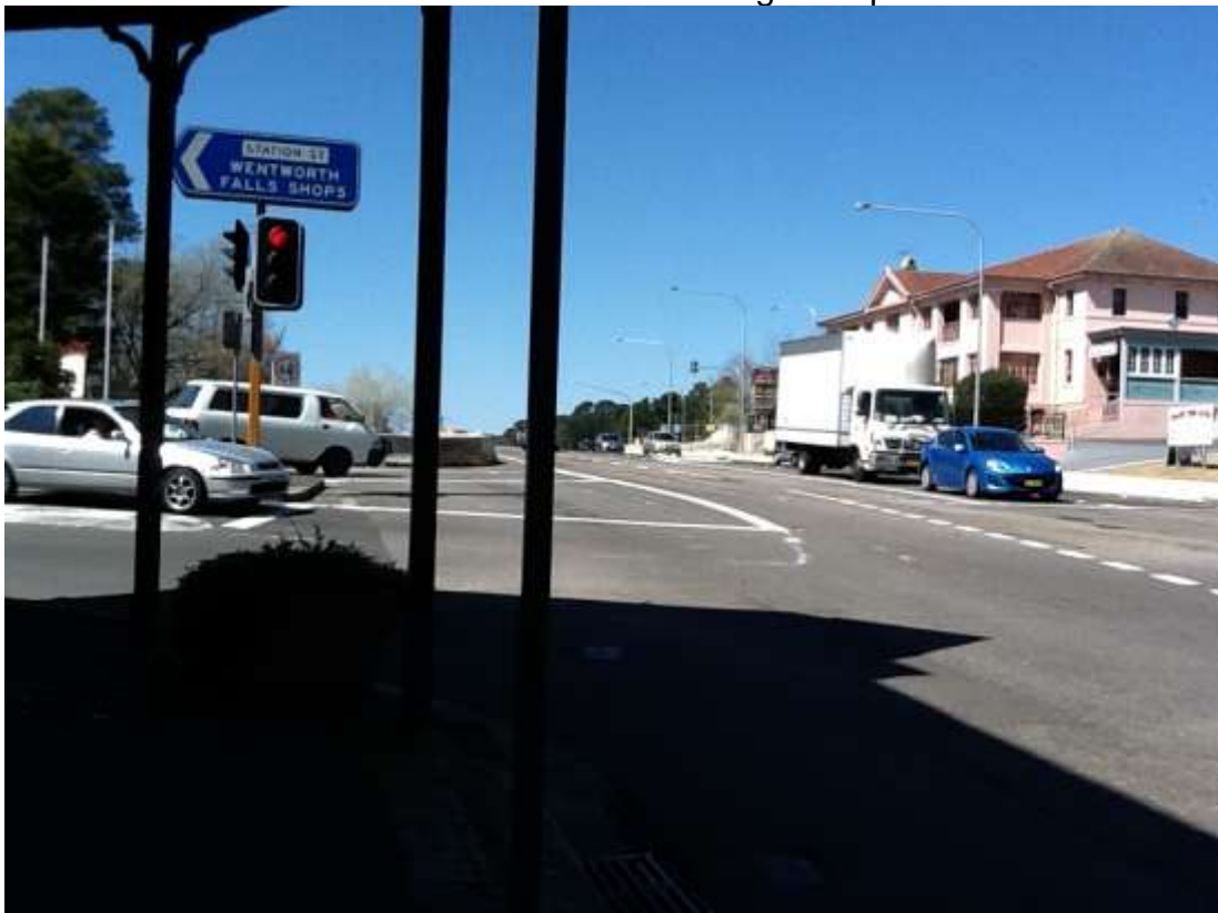
Intersection looking east to crest. The current upgrade ceases to the east of this intersection. There have been in the order of six major traffic incidents at this intersection in the last five years.
