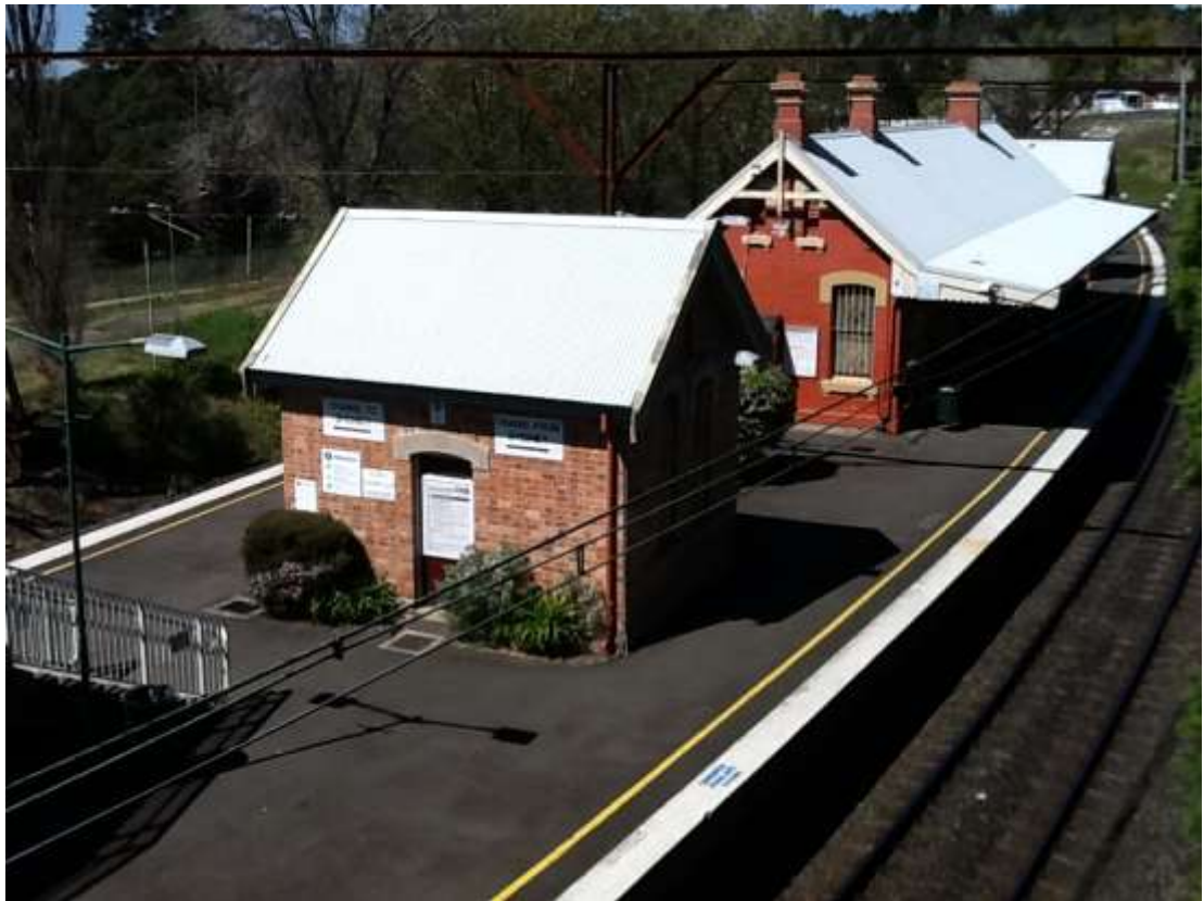
Wentworth Falls Rail Station
